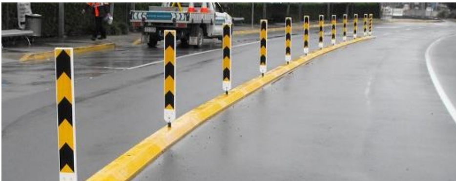
An example of temporary road kerb installation to direct traffic
