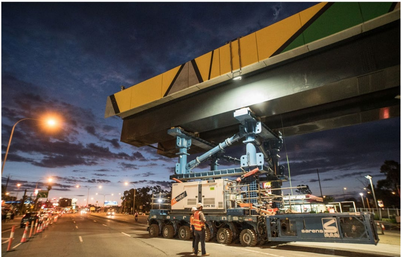
Darlington Upgrade Project – Overpass installation using SPMTs
